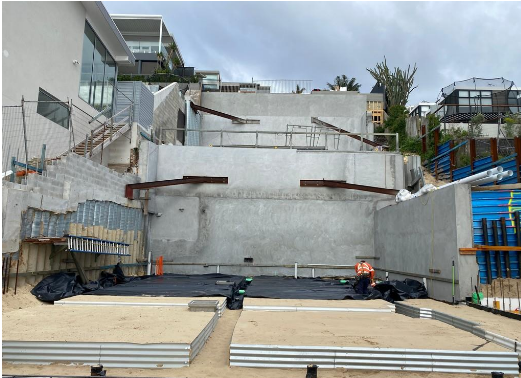
Figure 2: Photograph taken 9 December 2022. Since this date the concrete slab has been poured and formwork for levels above constructed. Reinforcing bracing to the walls is shown.
