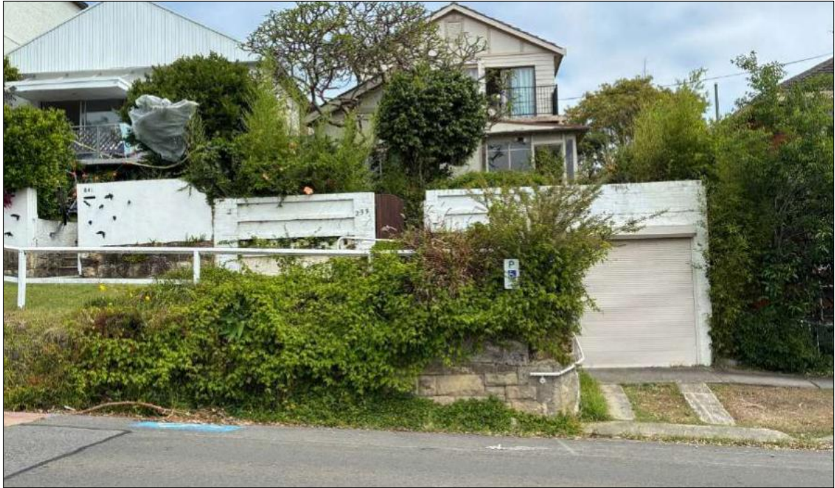
Figure 1: Existing dwelling (Source: Applicant's SEE)
