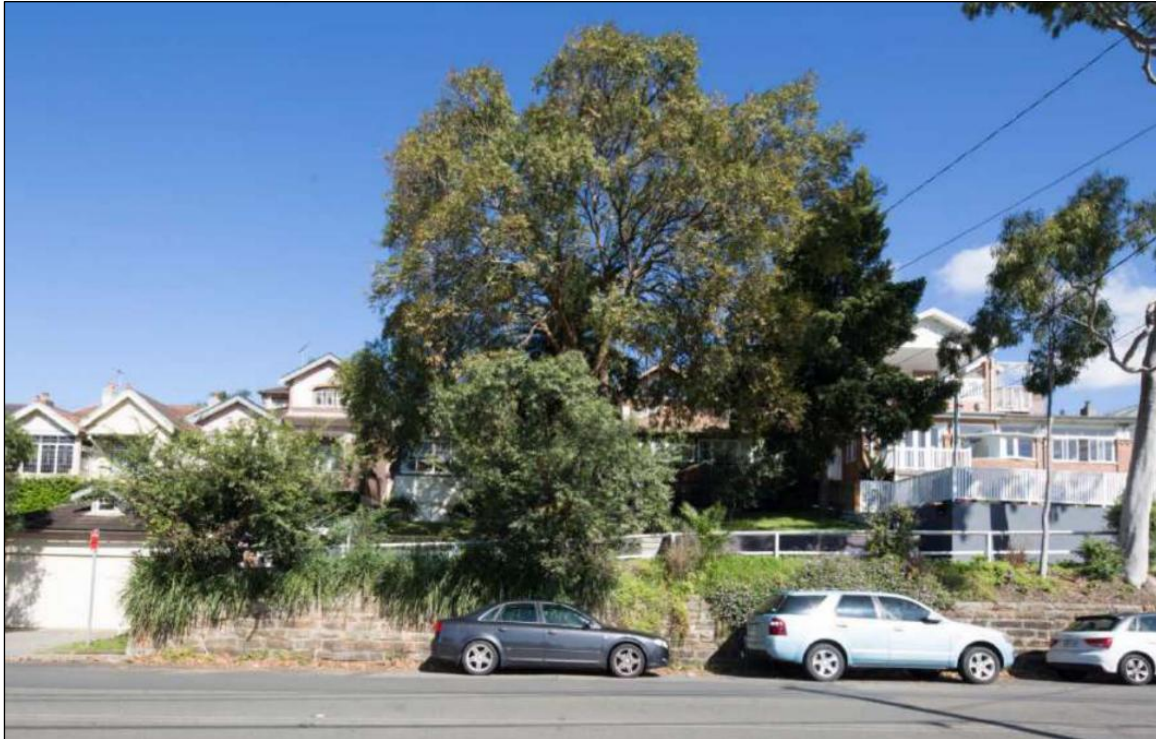
Figure 3: Existing sandstone retaining wall within Council's road reserve
