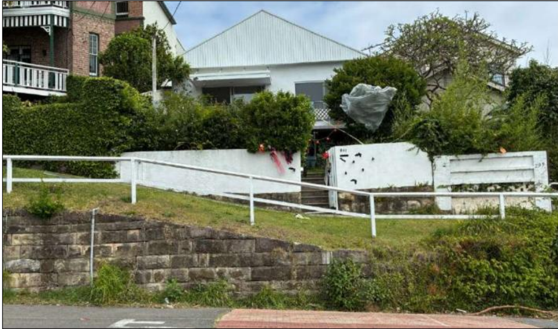
Figure 1: Existing dwelling (Source: Applicant's SEE)
