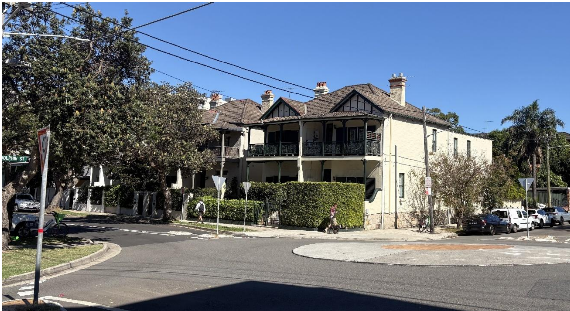
Figure 4: Photo of 90-92 Brook Street – taken from south west (Source: Council)
