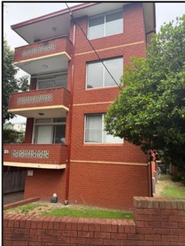
Photo 4: Adjoining flat building to the south at No. 76 St Marks Road.
