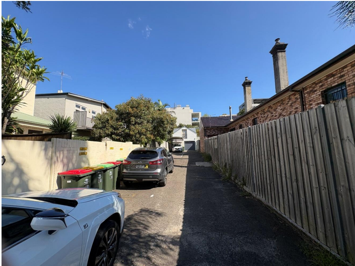
Figure 5: Photo of private lane at the rear of Brook Street terraces – subject site on right (Source: Council)
