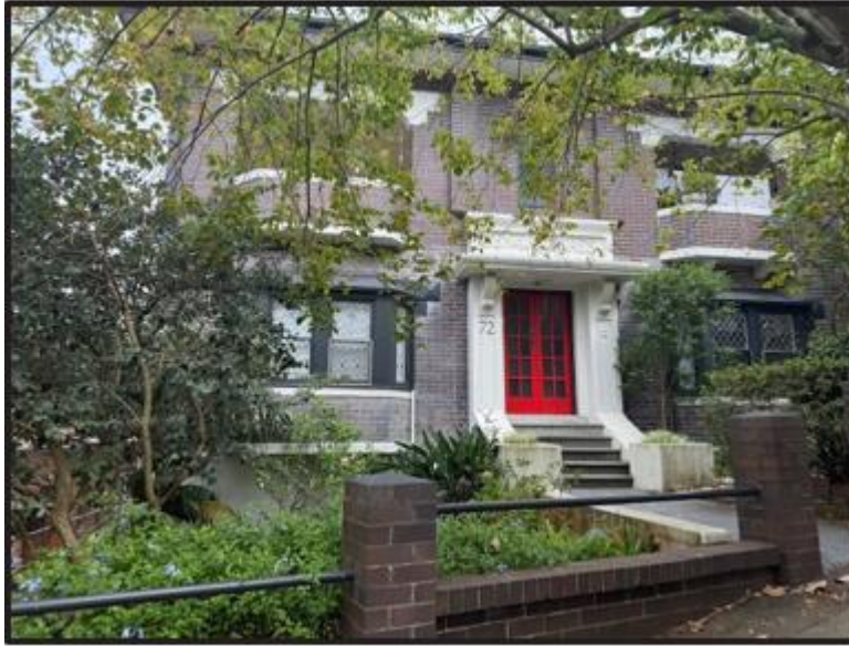
Photo 3: Adjoining flat building to the north at No. 72 St Marks Road
