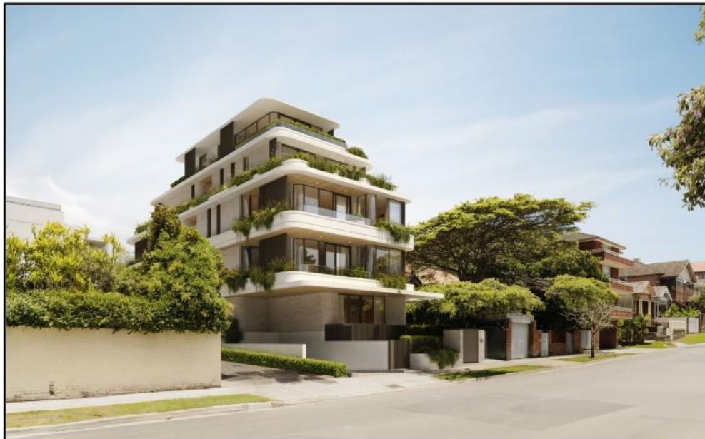
Figure 5: Extract of the photomontage demonstrating that the proposed development is compatible with the bulk and height of buildings along the streetscape
