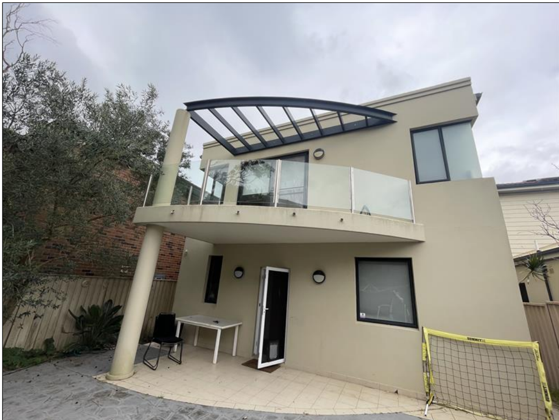
Figure 5: View from rear setback towards first floor rear facing balcony proposed to be squared off
