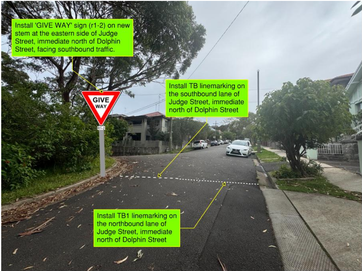
Figure 2: Street View – Intersection of Judge Street and Dolphin Street (Signs: SR-791558 and Lines: SR-791559)
