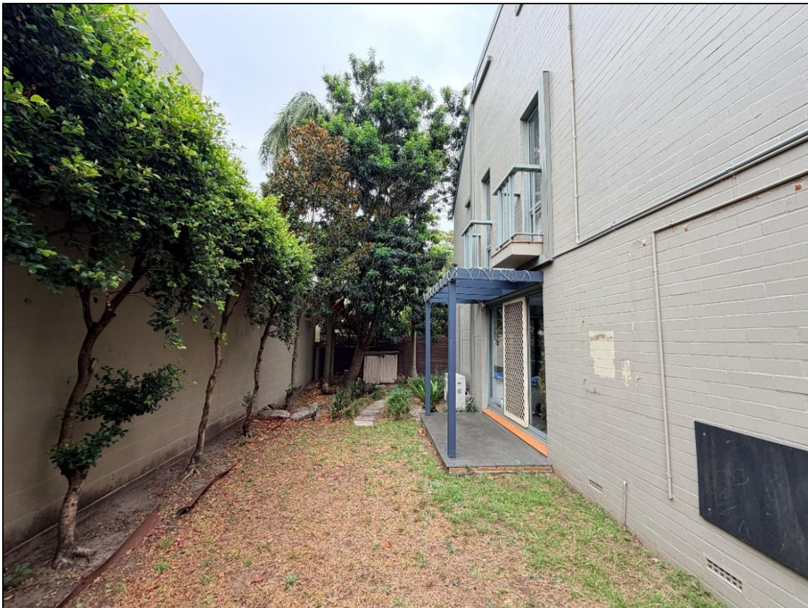
Figure 7. Courtyard subject to ground floor addition facing west (Source Council Officer).
