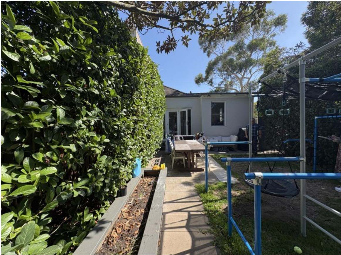
Figure 6: Existing rear elevation, viewed from southern (rear) boundary
