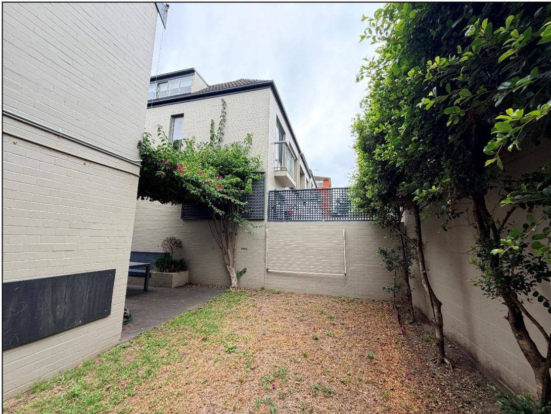
Figure 8. Remaining courtyard area (Source Council Officer).
