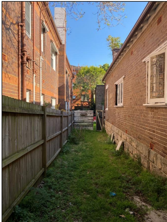
- Figure 37: Existing interface between development site and 31 Stanley Street (Source: Applicant)
