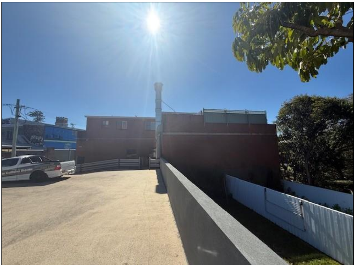
• Figure 3 – 1 Lingard Street Randwick adjoining car park (source: Assessing Officer)
