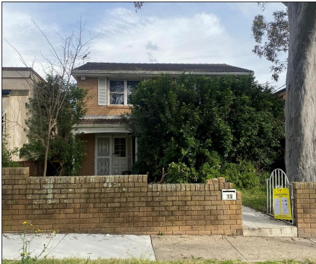
D. Figure 4: Existing building at 15 Strachan Street (Source: Council)
