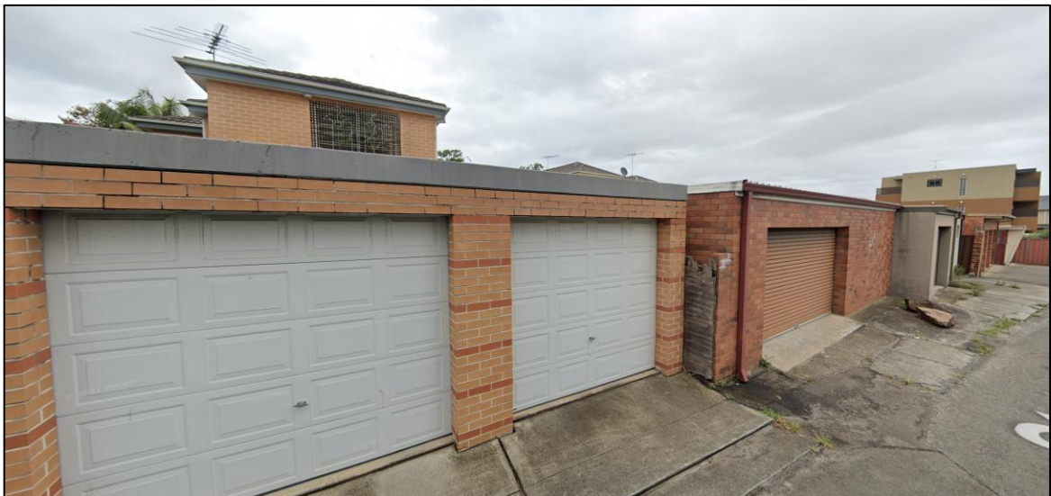
O. Figure 15: Garages of See Street Properties, which front Strachan Lane (Source: Google Maps)
