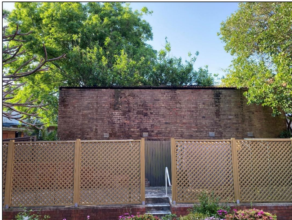
- Figure 8: Existing outbuilding as viewed from 42 Avoca Street (Source: Council)
