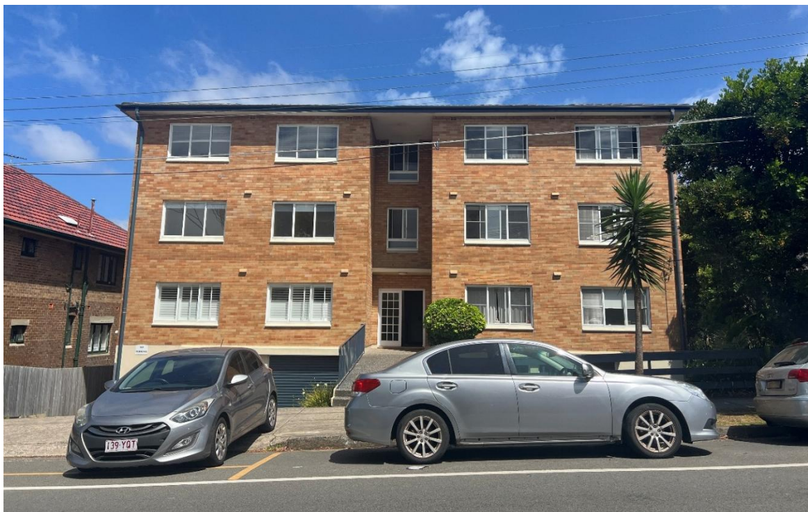
Figure 2: Subject Site viewed from Fern Street (Source: Council Officer)
