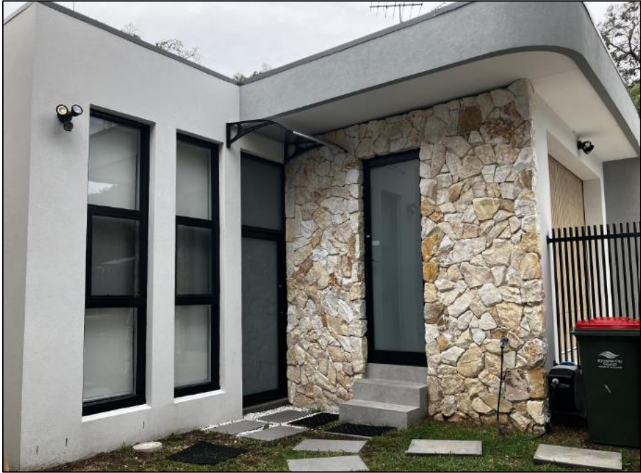
Figure 3: Outbuilding that is now being used for co-living rooms (Source: Council)
