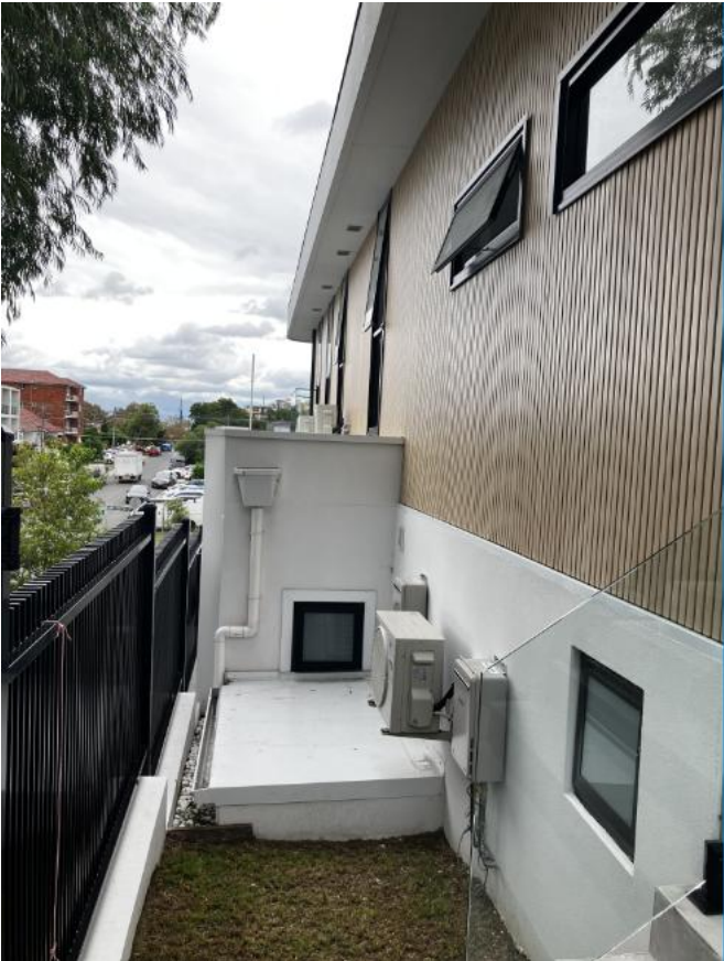
Figure 4: Southern Side Facade of 21 Forsyth Street (Source: Council)
