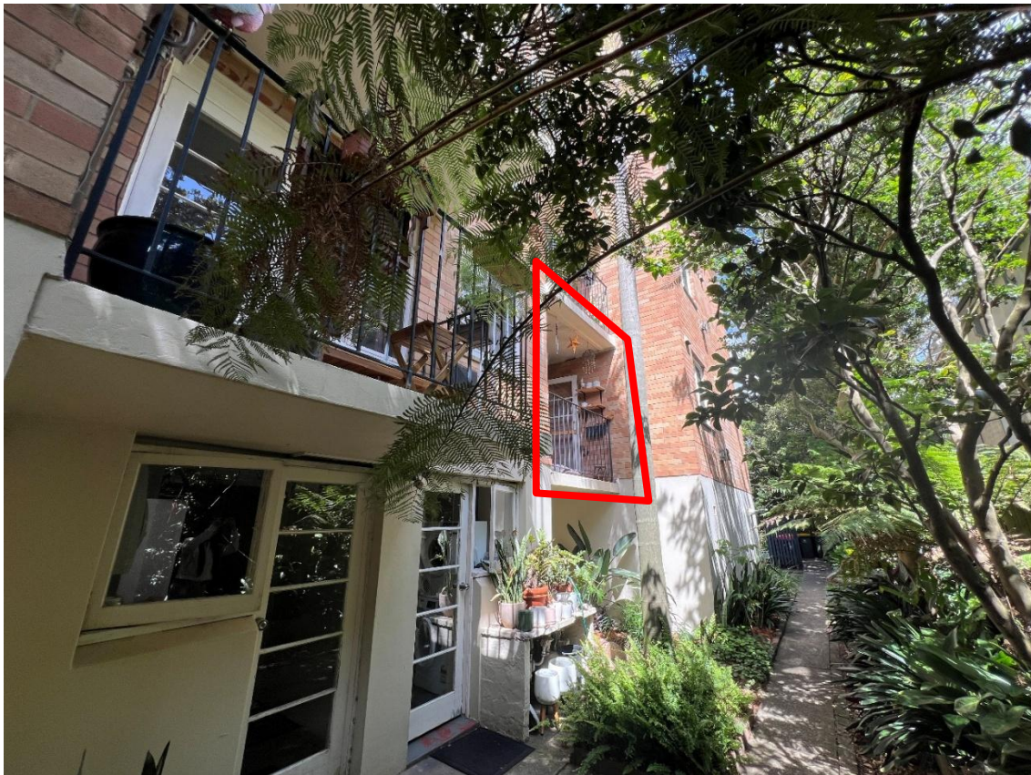
Figure 4: Existing balcony viewed from the northern side setback (Source: Council Officer)
