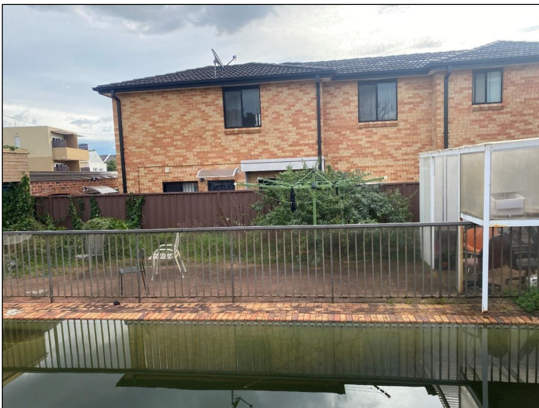
H. Figure 8: View from 17 Strachan Street towards 13 Strachan Street (Across 15) (Source: Council)
