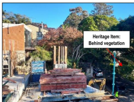
Photograph 1: The position of the heritage item in relation to the subject site, as viewed from the site looking northwest
