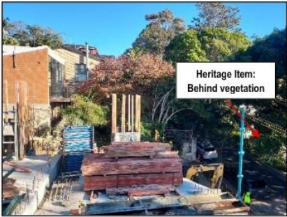
Photograph 1: The position of the heritage item in relation to the subject site, as viewed from the site looking northwest
