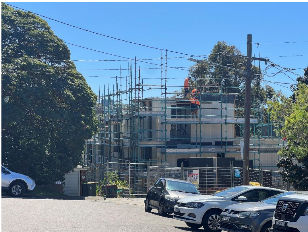
Figure 2. Subject site viewed from Heath Street (Source: Council Officer)
