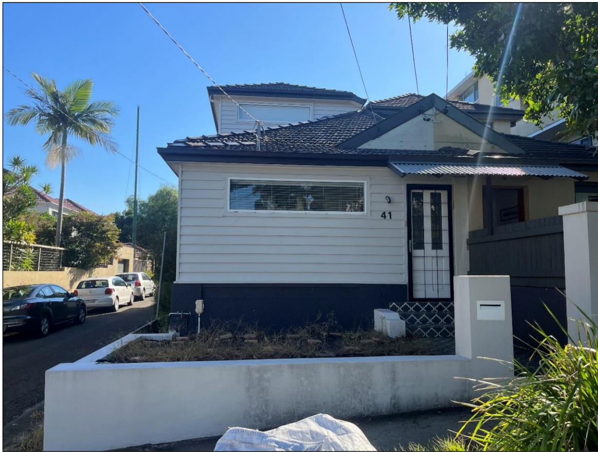
Figure 1: The front elevation of the subject site viewed from the footpath along Oberon Street.
