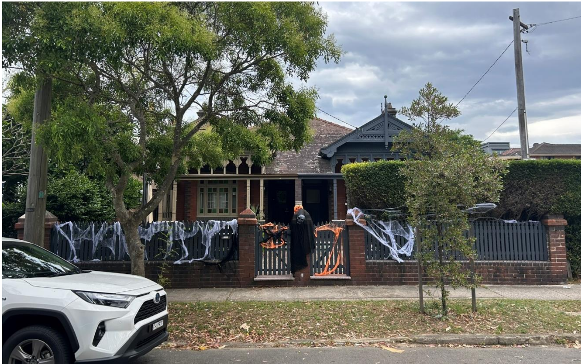
Figure 7: Semi-detached dwellings at 24-26 Abbotford St, viewed from Abbotford St (Source: Council officer)
