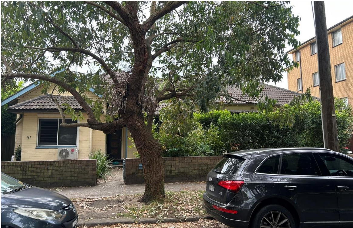
Figure 2: Existing development at Nos. 11-13, viewed from Abbotford St (Source: Council officer)
