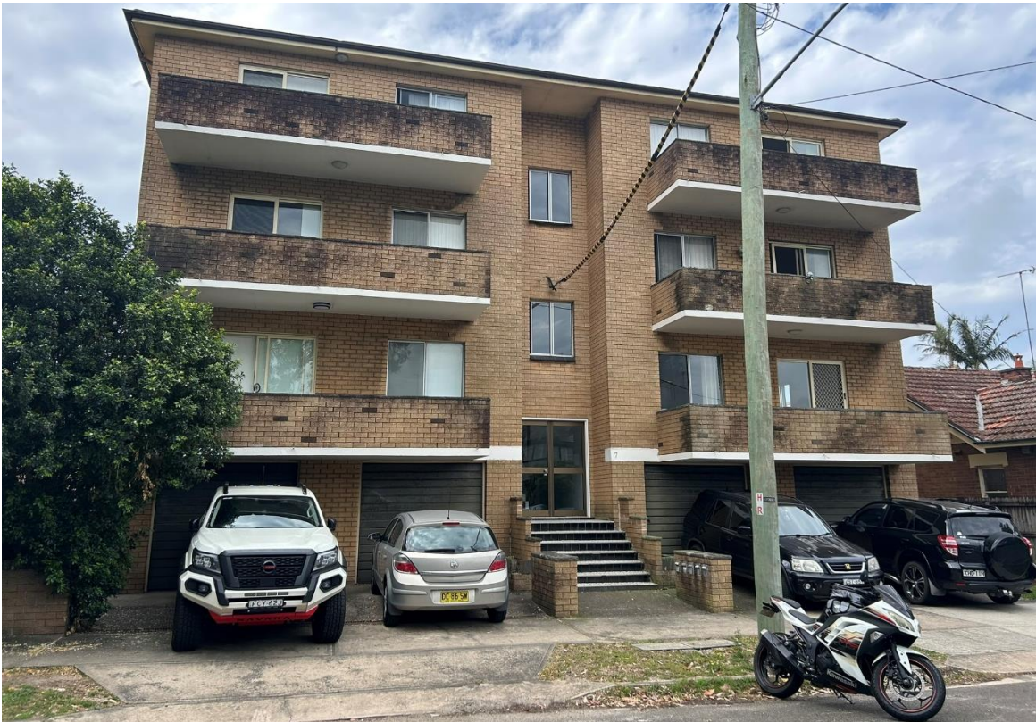
Figure 3: RFB at 7 Abbotford St, viewed from Abbotford St (Source: Council officer)
