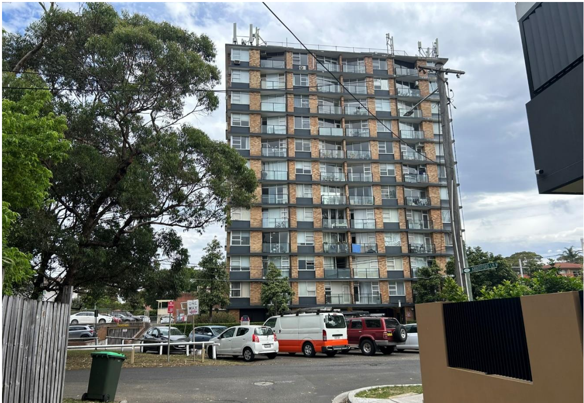
Figure 6: RFB at 56-62 Anzac Pde, viewed from Abbotford St (Source: Council officer)
