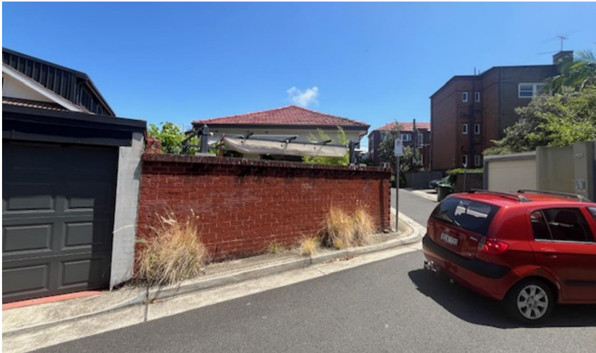
Figure 3: Rear of subject site, viewed from Division Lane (Source: Council officer)
