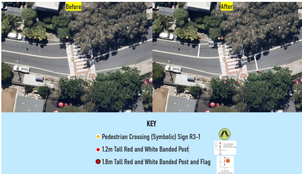
Figure 2. Cowper Street Before and After Improvements
