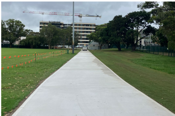
Concrete path – facing north
