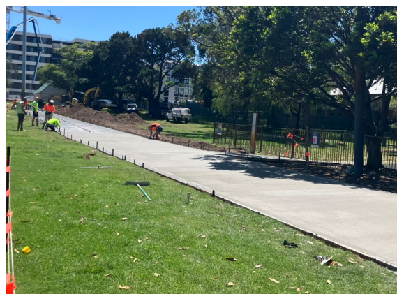
Concrete path concrete pour – facing north
