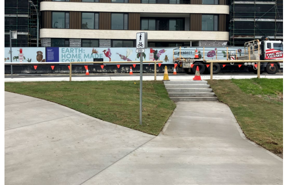
Stairs to Fennelly Street footpath – facing north
