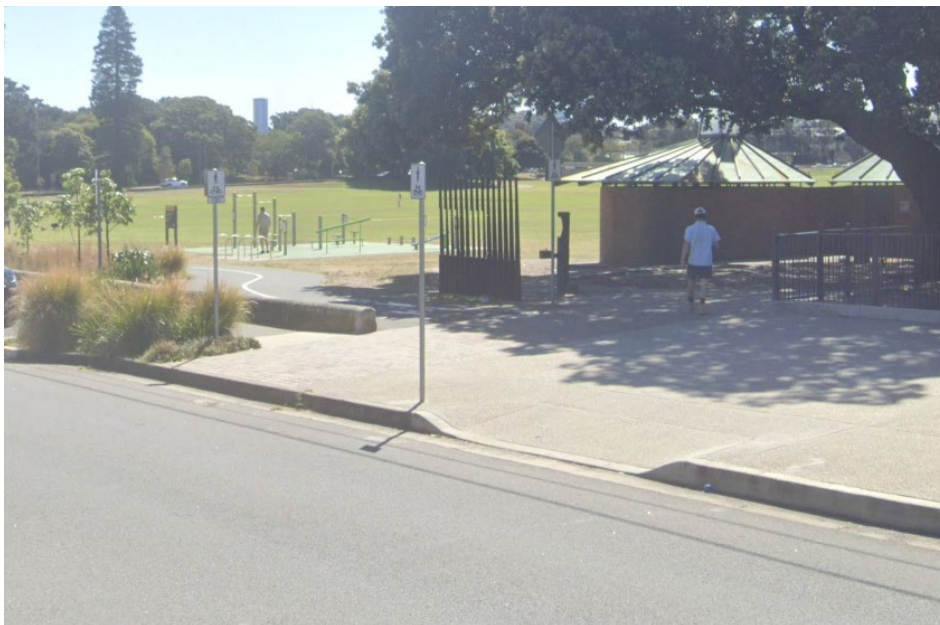
Kerb layback on the northern side of Darley Road, opposite of Market Street – facing south
