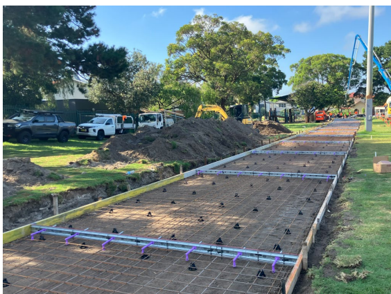
Concrete path form works – facing south
