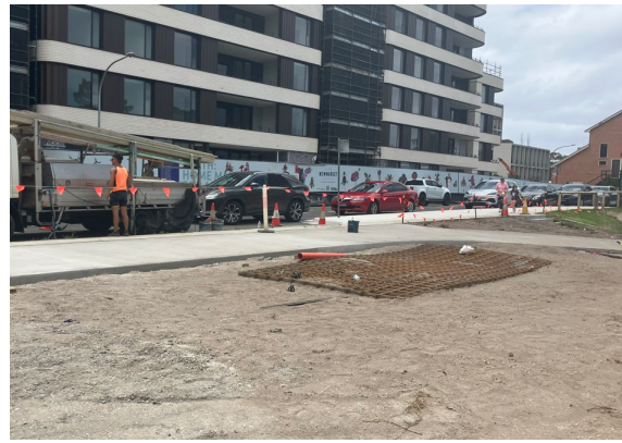
Fennelly Street concrete path expansion – facing north
