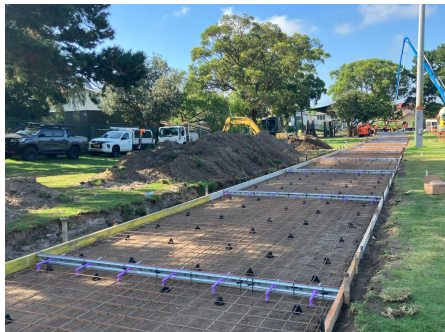
Concrete path form works – facing south
