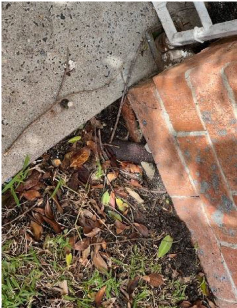
Tree roots inside fence and damage
