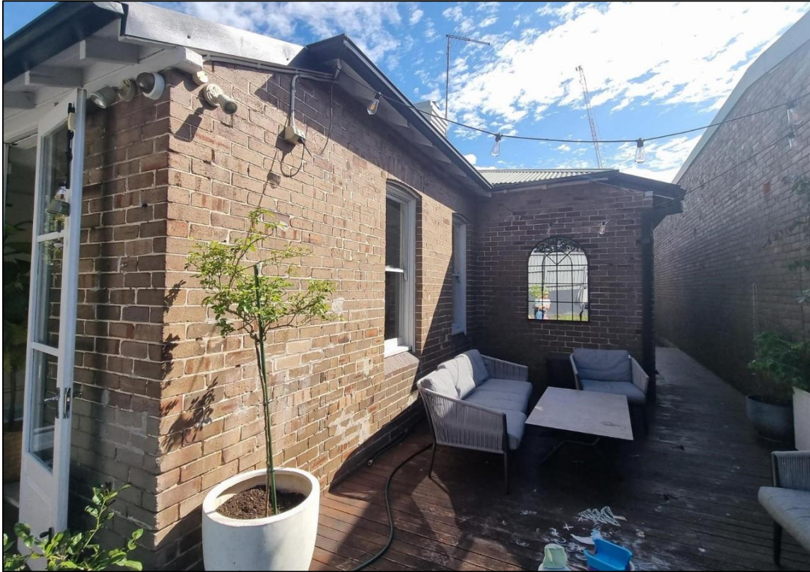
Figure 10. Original wall to the rear of the dwelling to be partially removed and replaced with new glass door openings.
