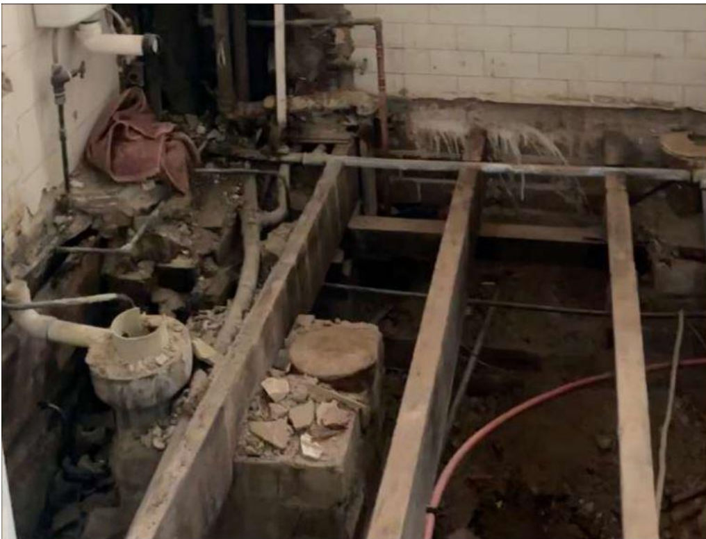
Figure 14: The bathroom floor was removed to facilitate emergency corrective maintenance as noted in the brief report prepared by County Road Plumbing Pty. Ltd. (Source: Weir Philips Heritage and Planning )
