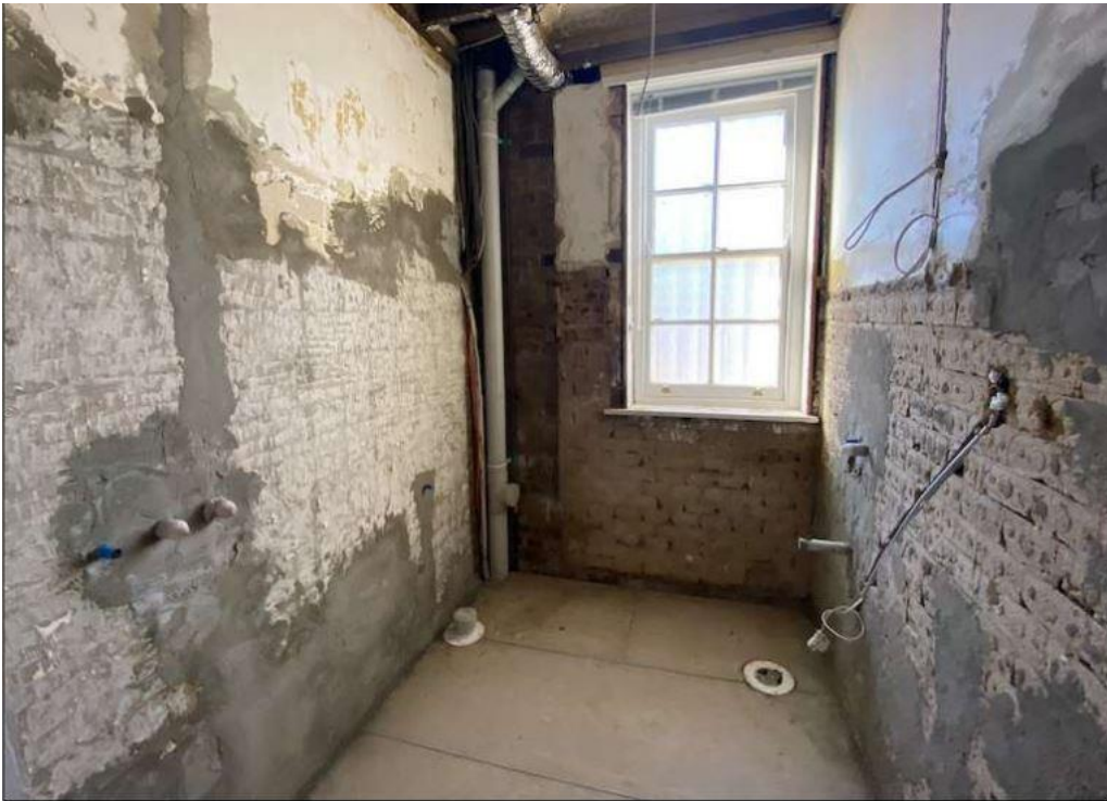
Figure 13: The bathroom has been striped, and a new fibre cement sub-floor has been installed on the original timber floor joists. (Source: Weir Philips Heritage and Planning )
