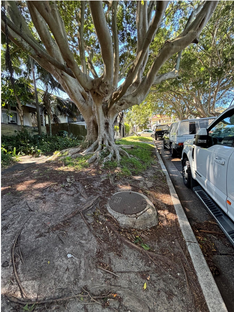
Photo 6 – Proximity of sewer main manhole
