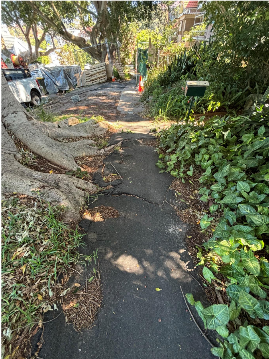
Photo 4 – Asphalt footpath – Tree root damage
