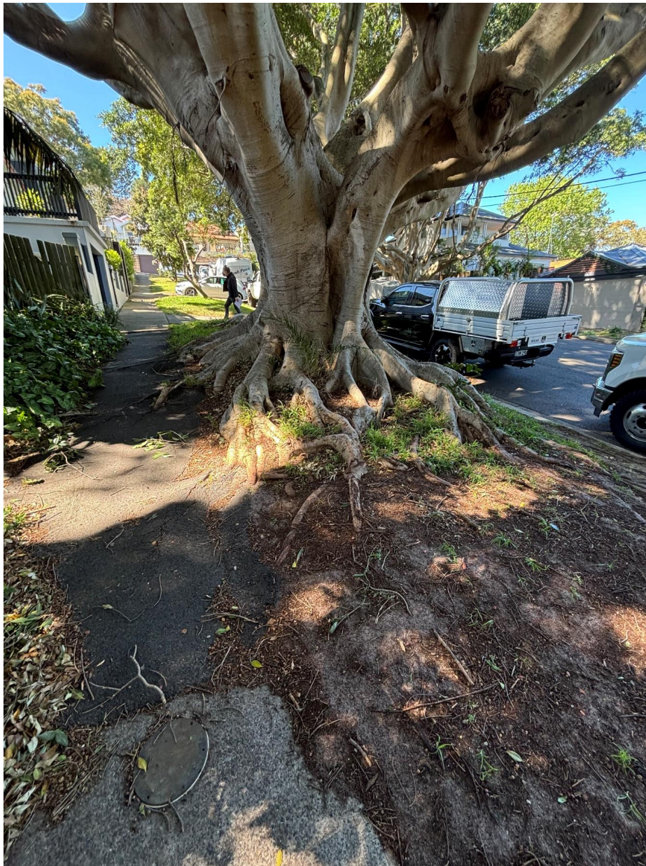
Photo 5 – Asphalt footpath – Tree root damage – Looking east
