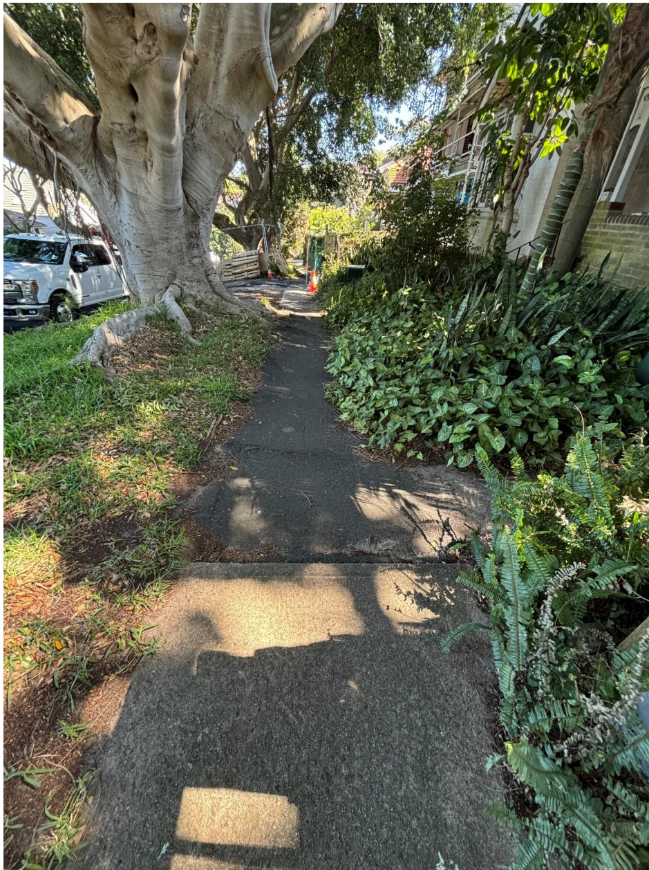
Photo 3 – Concrete footpath previously replaced with asphalt
