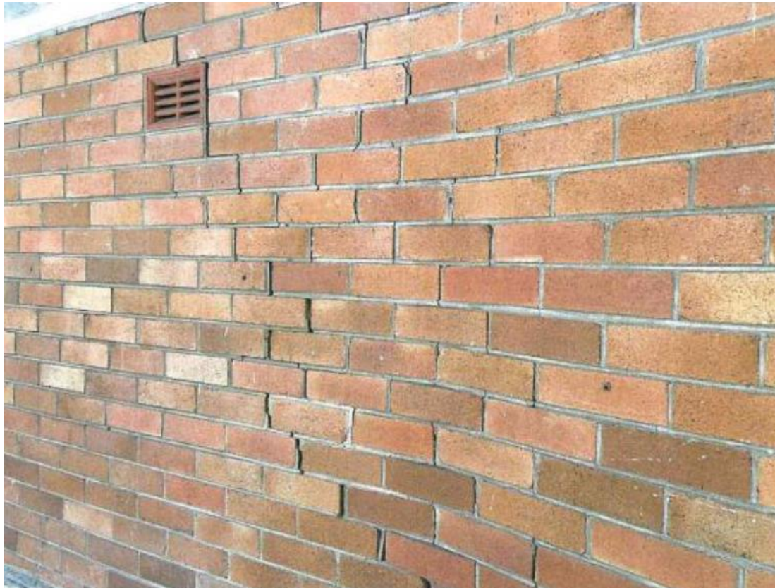
Figure 2: photo showing the cracking in the masonry wall (source: Town Planning Collective)
