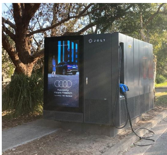
Figure 19: Photo of the Jolt EVCS on Beauchamp Road with the charging cable on the roadway (Source: Randwick City Council)
