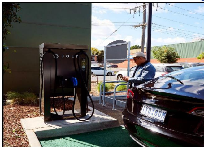
Figure 3. JOLT charging podium while not in use. Highlighting cable retraction mechanism and no trailing cables
