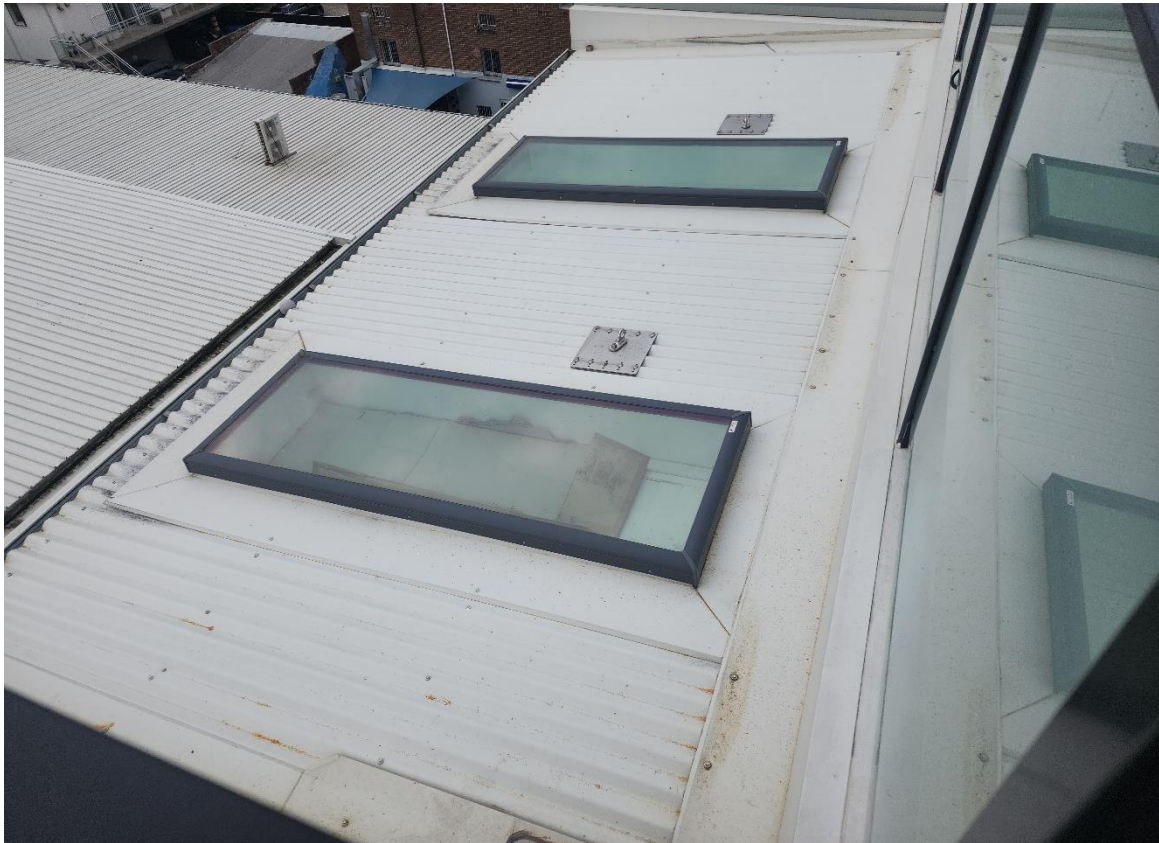
Figure 6: Roof and skylight enclosure of the former terrace to sunrooms
