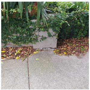
Photo 14. Cracked pillar on nearby fence which may have been caused by root pressure.
