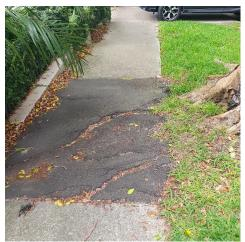
Photo 13. Repaired section of footpath that is now lifted by root pressure.
