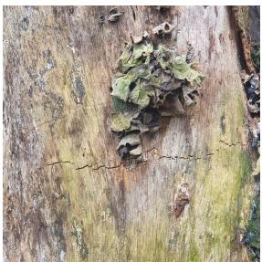
Photo 11. Wood checking crack lower trunk.
