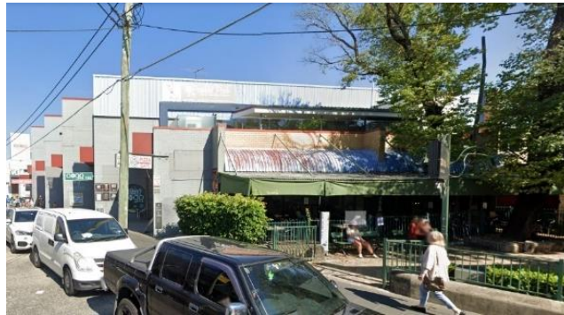
Figure 9: Poor interface between shopping centre and June Moore Place
