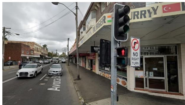
Figure 10: Dilapidated state of the traditional night-time zone
