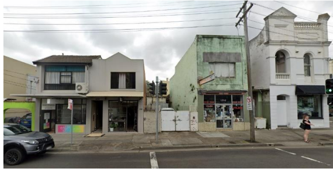
Figure 8: Dilapidated shopfronts and heritage facades on Avoca Street
