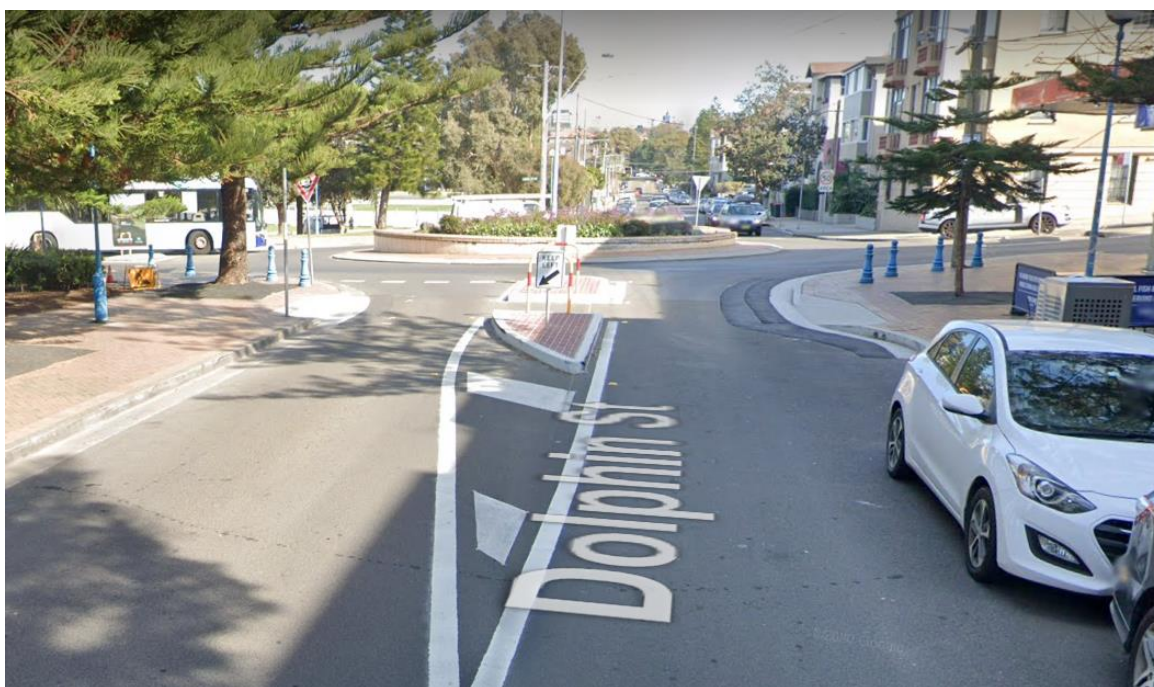
Pedestrian refuge which replaced the previous painted splitter island – note additional kerb nib as well
