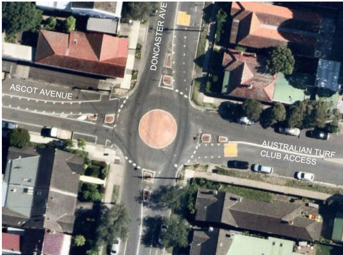
Figure 1 – Doncaster Avenue and Ascot Street roundabout intersection pre-construction
