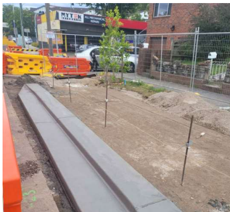
Kerbs for separated cycleway - Doncaster Avenue, south of Anzac Parade, facing south
