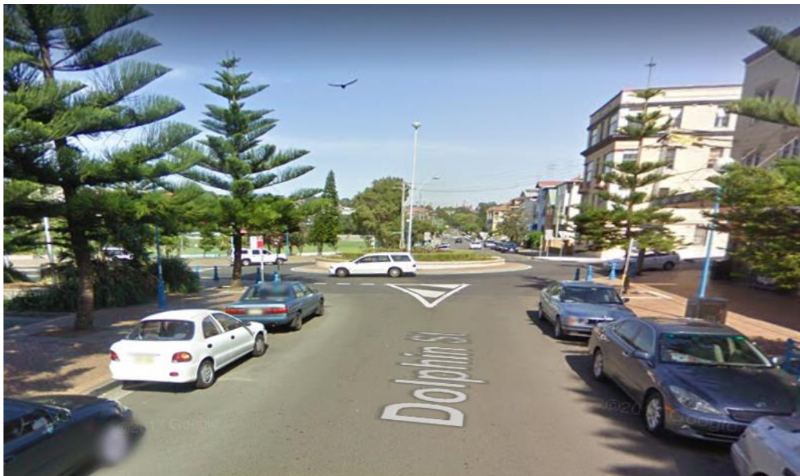
Previously existing painted splitter island on the westbound Dolphin Street approach to roundabout
