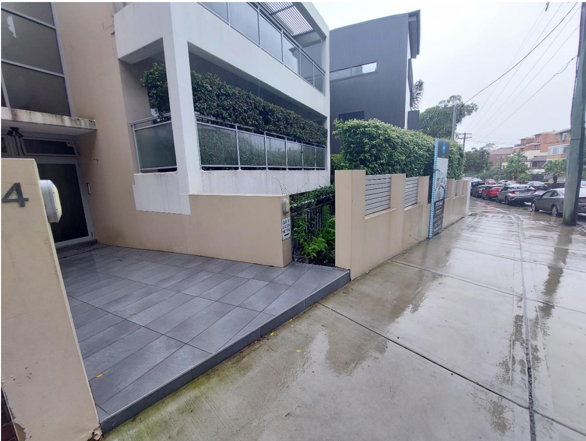
Figure 4 – View from Coogee Bay Road
