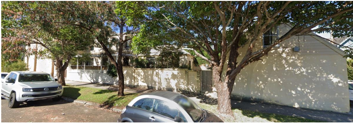
Figure 3: Photo of the side of the entire subject site including the garage at the rear of Douglas Street frontage at No. 2 Bishops Avenue, Randwick.
