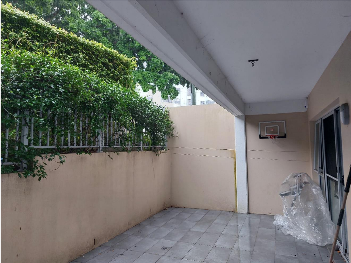
Figure 3 - Existing lower terrace (looking north)
