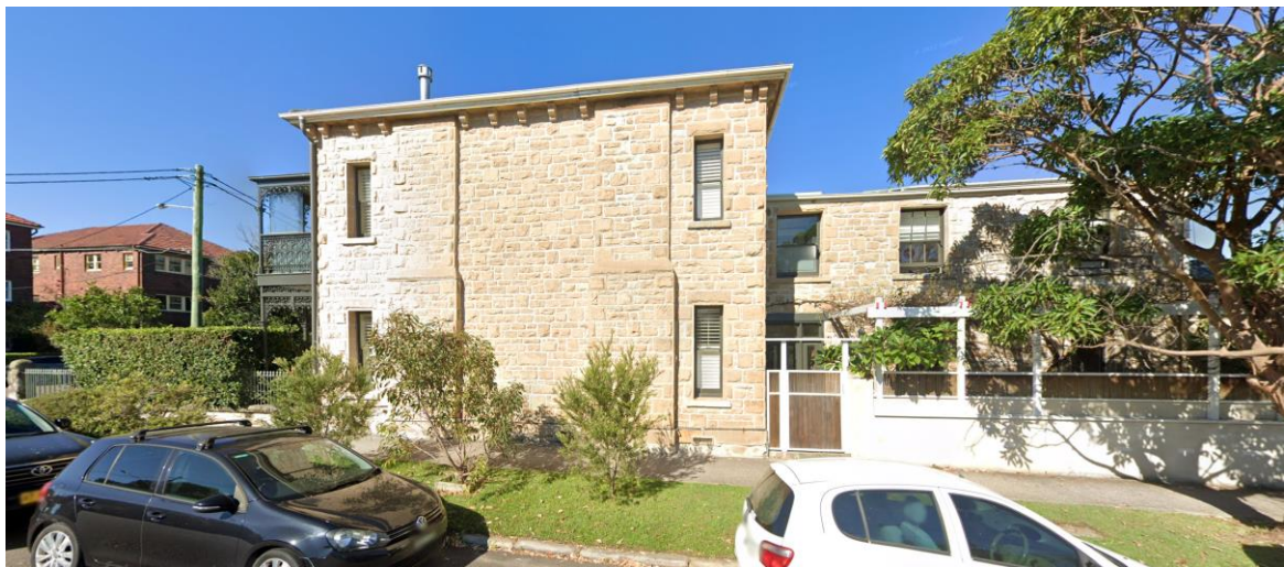
Figure 2: Photo of the side of the subject site at the Douglas Street frontage at No. 2 Bishops Avenue, Randwick.
