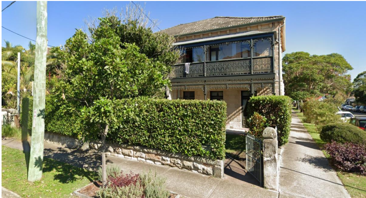
Figure 1: Photo of the front of the subject site at No. 2 Bishops Avenue, Randwick.
