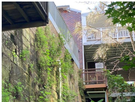
Figure 15. Partial view of the rockface and sandstone blocks forming the retaining wall running east-west through the middle of the subject site.
