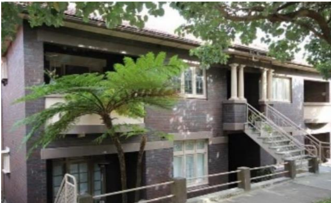
Image 2: General view of the main façade, looking westwards
