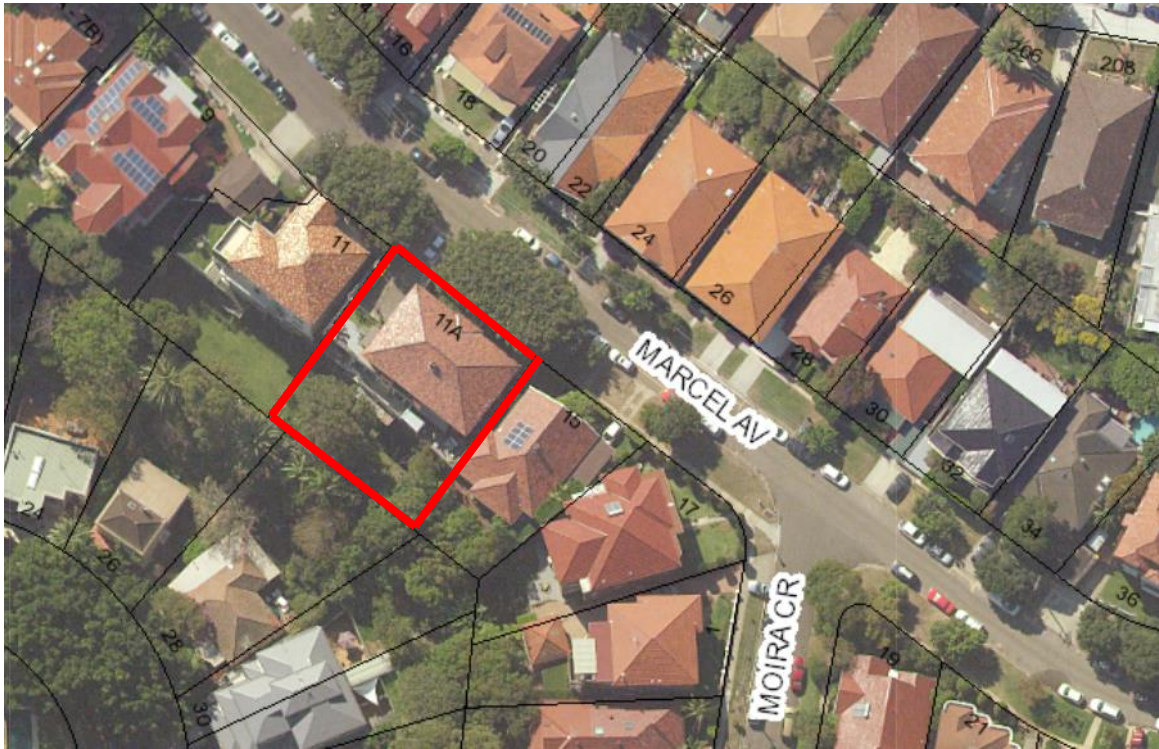
Image 1: Aerial photograph of the subject property (11A Marcel Avenue, Coogee) outlined in 'red'.
